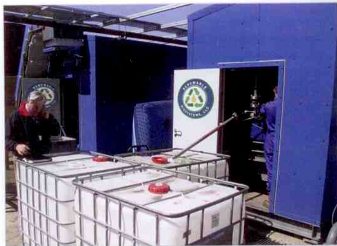
Oil totes are filled and sent to their destination, such as a nearby biodiesel plant for further cleaning and processing into fuel.
